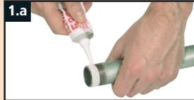
1.a Use a threaded paste sealant, we recommend LOCTITE 5331 or...
