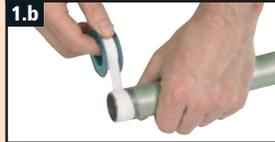
1.b Use a teflon tape sealant. The right sealant for threaded joints is non-hardening, compatible with plastic and doesn't add slipperiness to encourage over-torquing.
