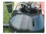
Fix wire clip into opposing holes on body sides. Ensure the wire runs parallel with the pipe as shown in the image. Screw wire clip holders into the holes provided.
