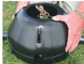
Locate body on skid base and push firmly down to engage grip lugs.
