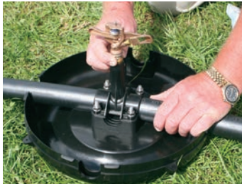
Screw sprinkler into sprinkler riser.
