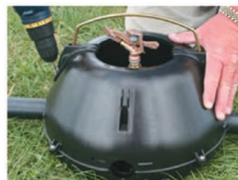
Screw wire clip holders into the holes provided.
