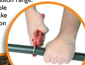
1. Cut the pipe with pipe cutters, knife or saw. Ensure a square cut of pipe ends. Clean burrs from pipe ends. Keep the pipe end clean and as free of scratches and imperfections as possible.
