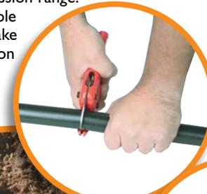
1. Cut the pipe with pipe cutters, knife or saw. Ensure a square cut of pipe ends. Clean burrs from pipe ends. Keep the pipe end clean and as free of scratches and imperfections as possible.
