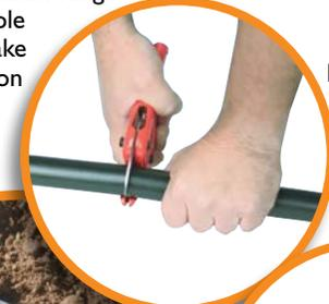
1. Cut the pipe with pipe cutters, knife or saw. Ensure a square cut of pipe ends. Clean burrs from pipe ends. Keep the pipe end clean and as free of scratches and imperfections as possible.
